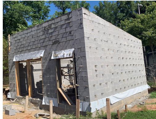
CSK- Storage CMU installation complete
